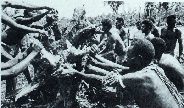
Numerous massive tree stumps were dug out and moved by hand to clear the airstrip which opened Niksek to help from the outside world.
